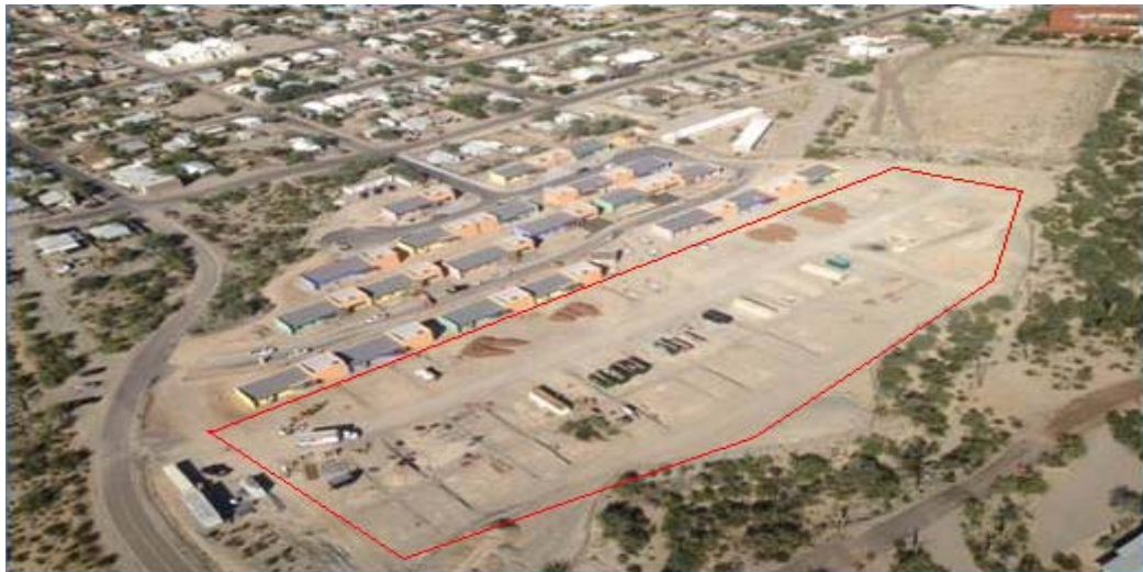
Figure 1: Land and CBP-built Housing in Ajo, Arizona
